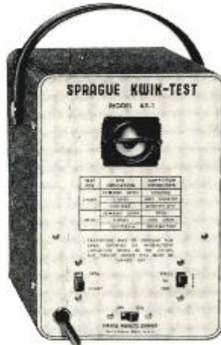
Sprague "Kwik-Test" capacitor checker.
